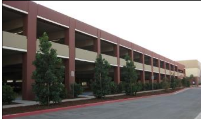
The Fremont parking structure, which has been under construction for a little over a year, opened on July 1st. The new structure has a total of 762 spaces.
