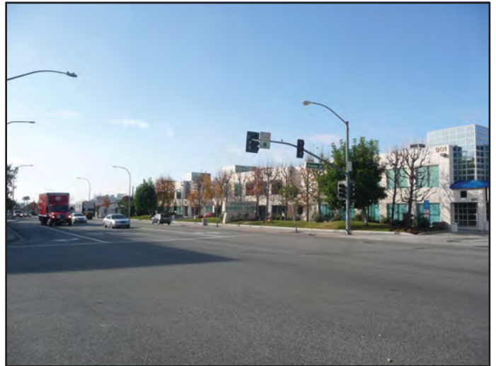
View 40: View looking southwest on the corner of Orange Street and Fremont Avenue of existing office buildings adjacent to the northwestern portion of the Project Site.
