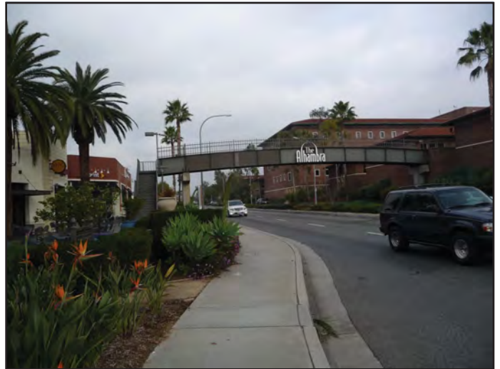
View 20: View looking northeast on Fremont Avenue of existing structure and pedestrian bridge adjacent to the southwestern portion of the Project Site.
