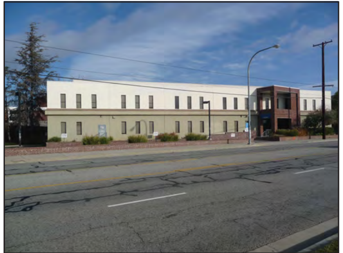
View 4: View looking northeast on Mission Road of the existing structure on the southern portion of the Project Site.
