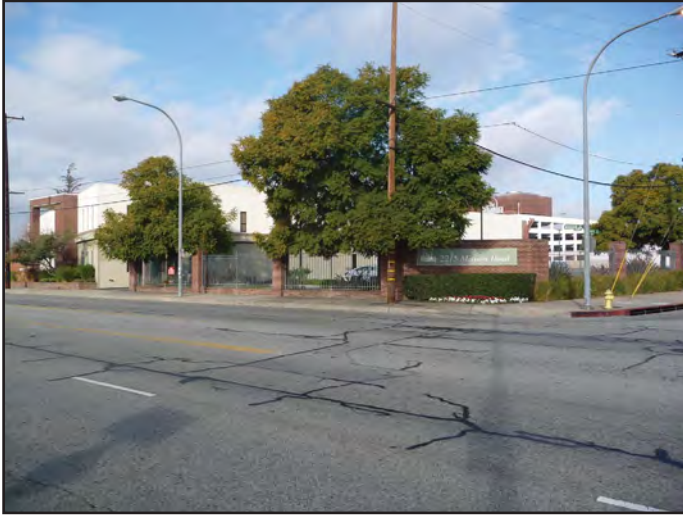
View 5: View looking northwest on the intersection of Mission Road and Date Avenue of the existing structures on the southeastern portion of the Project Site.
