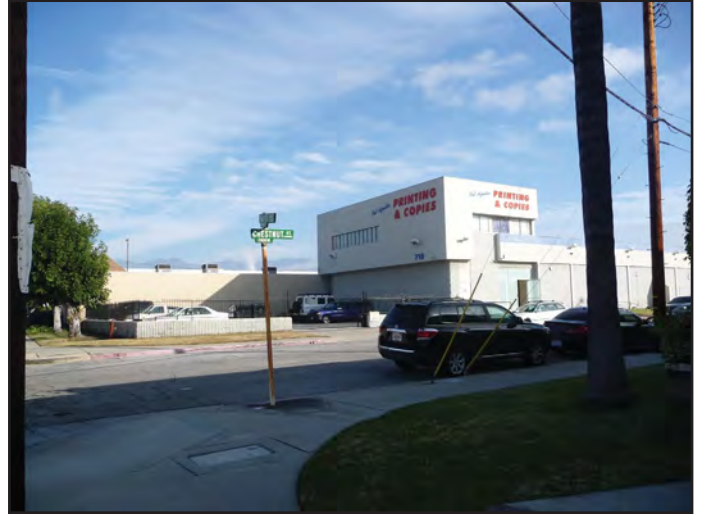
View 34: View looking northeast on the corner of Date Avenue and Chestnut Street of existing office buildings adjacent to the eastern portion of the Project Site.
