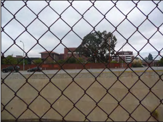
View 45: View looking north on Front Street of the existing structures on the southern portion of the Project Site.
