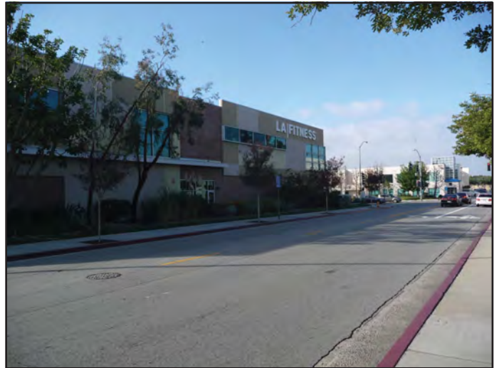
View 16: View looking southwest on Orange Avenue of existing structure adjacent to the northwestern portion of the Project Site.
