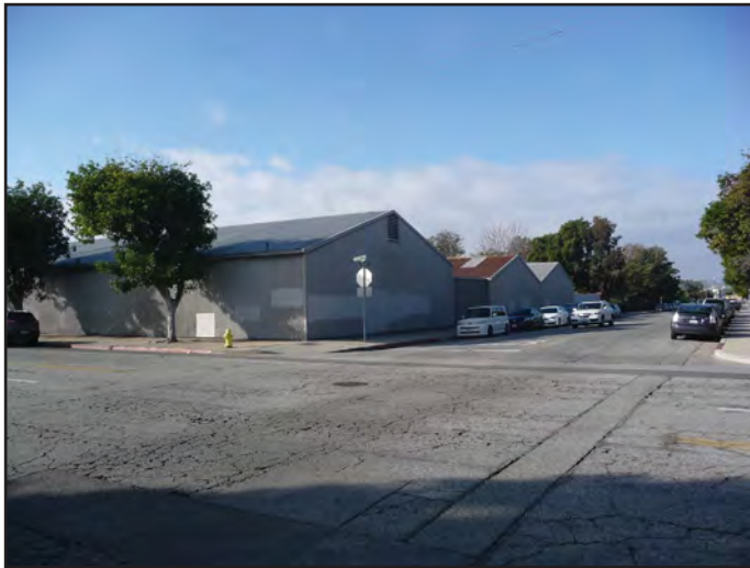
View 11: View looking southwest on the intersection of Date Avenue and Orange Avenue of the existing structures on the northeastern portion of the Project Site.
