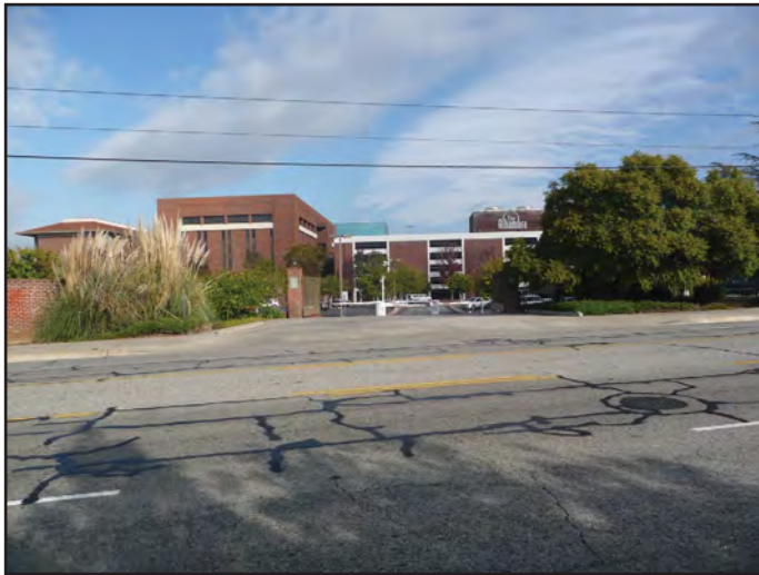
View 3: View looking north on Mission Road of the existing structures on the southern portion of the Project Site.
