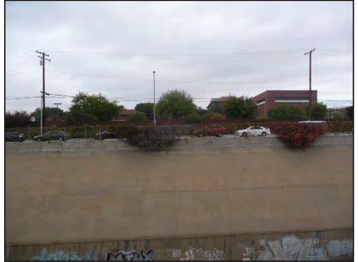
View 46: View looking north on Front Street of the existing structures on the southern portion of the Project Site.
