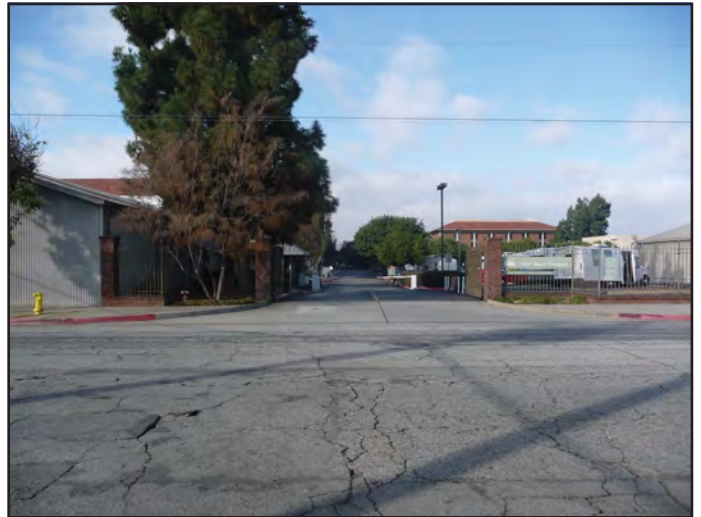
View 8: View looking west on Date Avenue of vehicle entryway and existing structures on the eastern portion of the Project Site.
