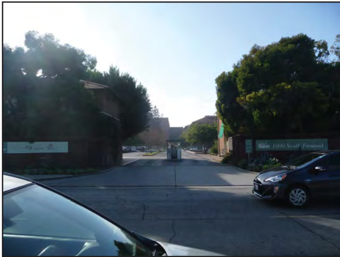
View 15: View looking south on Orange Avenue of vehicle entryway and existing structures on the northern portion of the Project Site.
