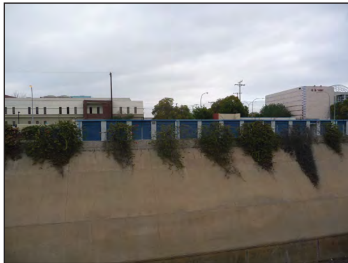
View 47: View looking northeast on Front Street of the existing structures on the southern portion of the Project Site.
