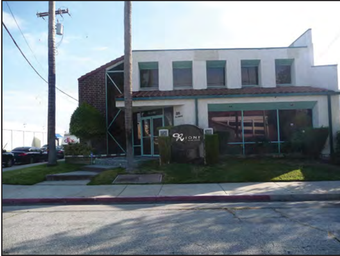
View 33: View looking east on the corner of Date Avenue and Chestnut Street of existing office building adjacent to the eastern portion of the Project Site.
