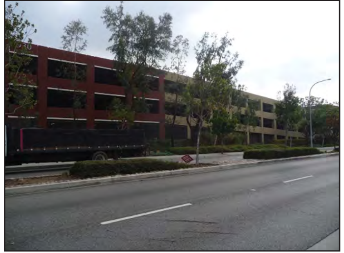
View 18: View looking southeast on Fremont Avenue of existing parking lot adjacent to the northwestern portion of the Project Site.
