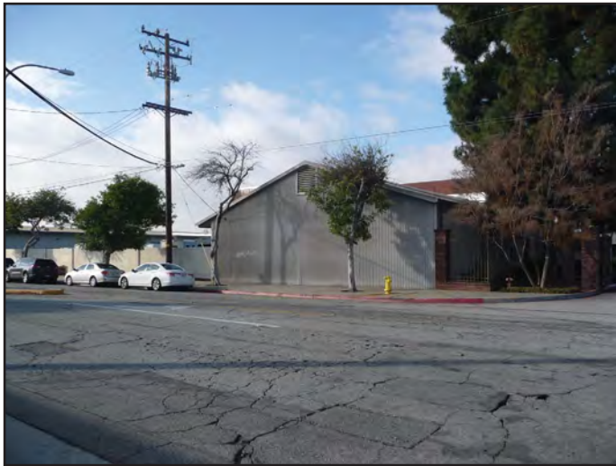
View 7: View looking southwest on Date Avenue of the existing structures on the eastern portion of the Project Site.
