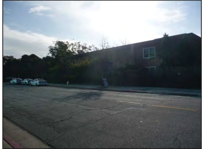
View 14: View looking southeast on Orange Avenue of existing structures on the northern portion of the Project Site.
