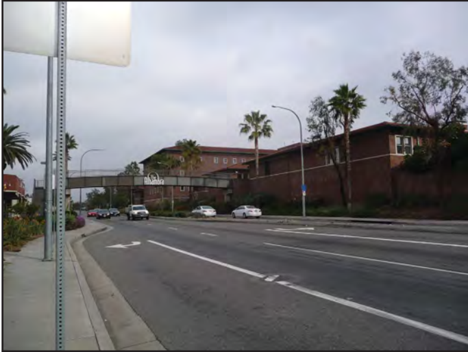
View 21: View looking northeast on Fremont Avenue of existing structure and pedestrian bridge adjacent to the southwestern portion of the Project Site.
